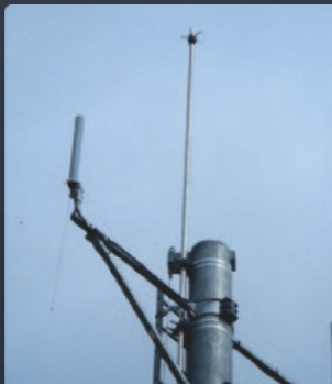
ESE air terminal in extreme climatic conditions
