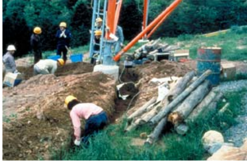
Excavation for SAN-EARTH Grounding
