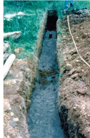
Laying SAN-EARTH M5C
