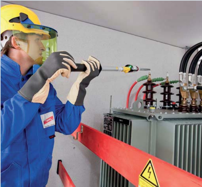
PHE III ZK voltage detector used in an indoor switchgear installation
