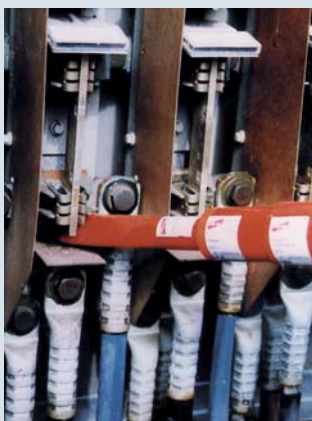
Chamfered flat cleaning head in use
