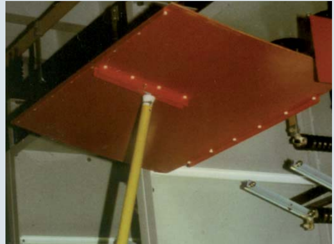
Inserting an insulating protective shutter of type A3
