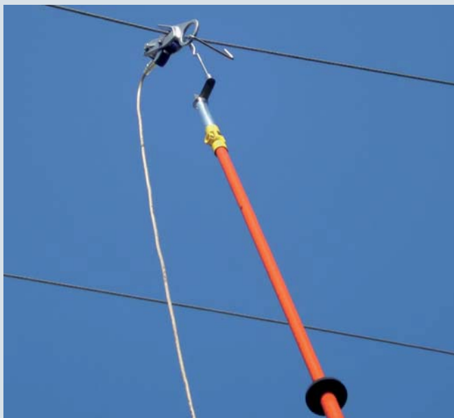
Removal of a phase clamp using a single-pole coupling aid
