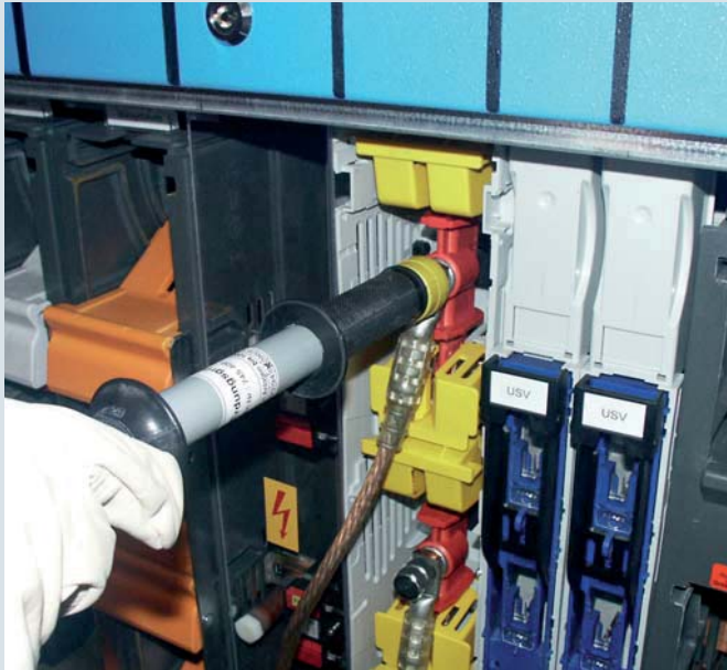
Attaching a partly insulated earthing and short-circuiting device using an earthing handle of type TI
