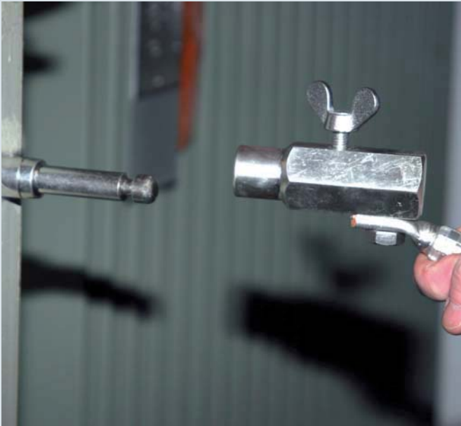
Fixed earthing point with ring groove and earth bushing
