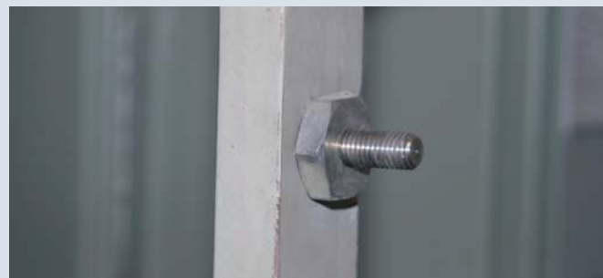
Earth connector with M12 threaded pin screwed to an earthed part of an installation
