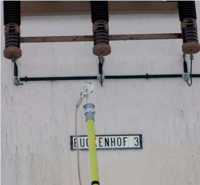
Rigid ball head cap with long shaft and earthing stick
