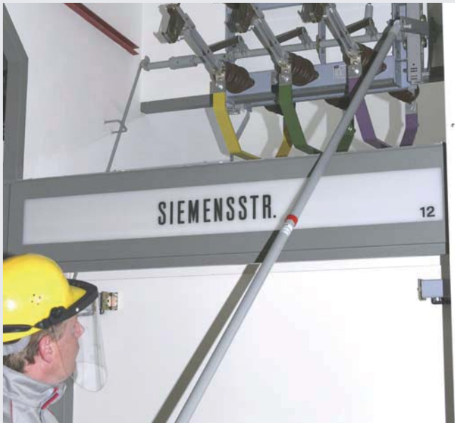
Switching a disconnector by means of an SCS switching stick
