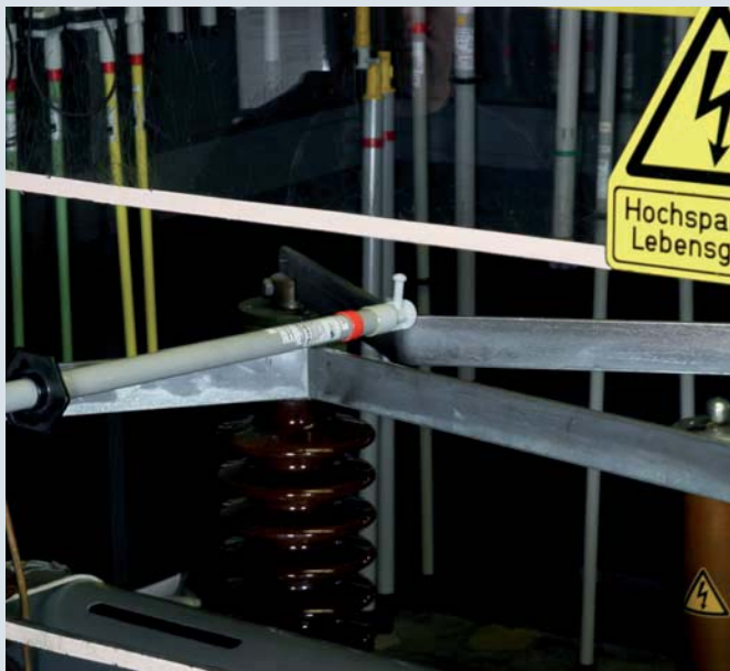
Testing a switchgear installation for protection against bridging
