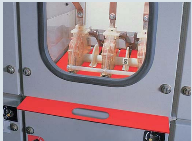
Inserting an insulating protective shutter of type A4
