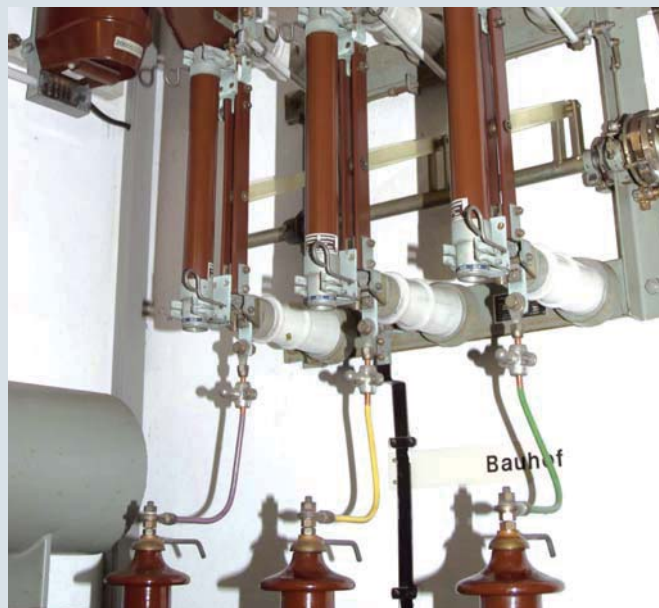
Fixed ball point attached to the round copper conductor of a switchgear installation
