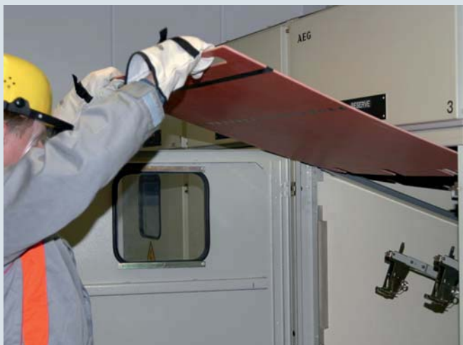
Inserting an insulating protective shutter of type A1
