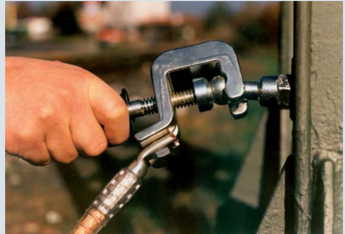
Universal clamp mounted on the fixed ball point of a steel tower
