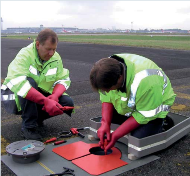
Replacement of a faulty illuminant (airport lighting system) at a runway
