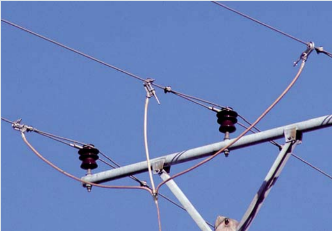
Phase screw clamps used on an overhead line
