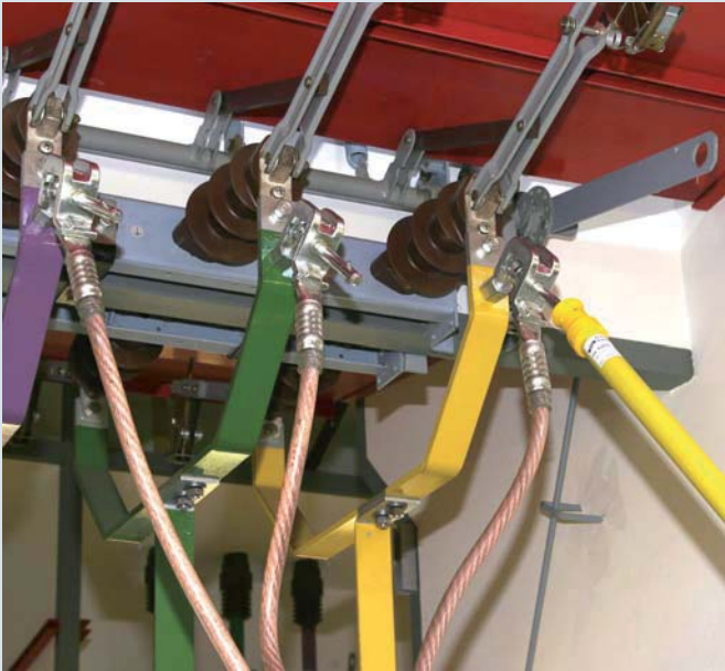
Earthing stick used for attaching an earthing and short-circuiting device to an installation
