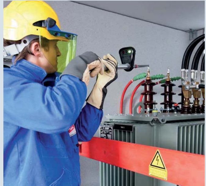
PHE voltage detector with visual indicator used on a switchgear installation
