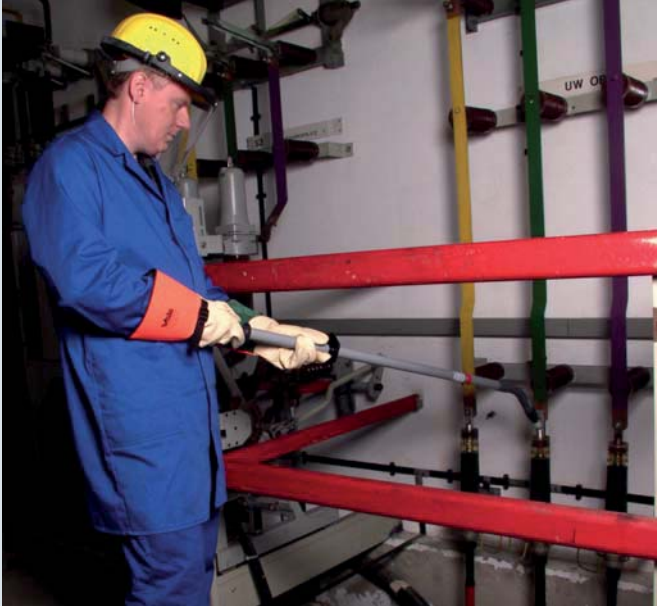
Loosening the locking screw using the MS insulated screw driver
