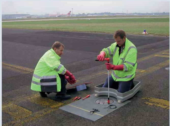
The insulating extension is used as insulating intermediate section when attaching the illuminant.
