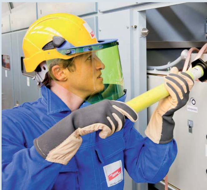
Attaching an earthing and short-circuiting device using the required personal protective equipment
