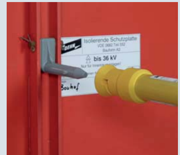
Inserting an insulating protective shutter of type A3
