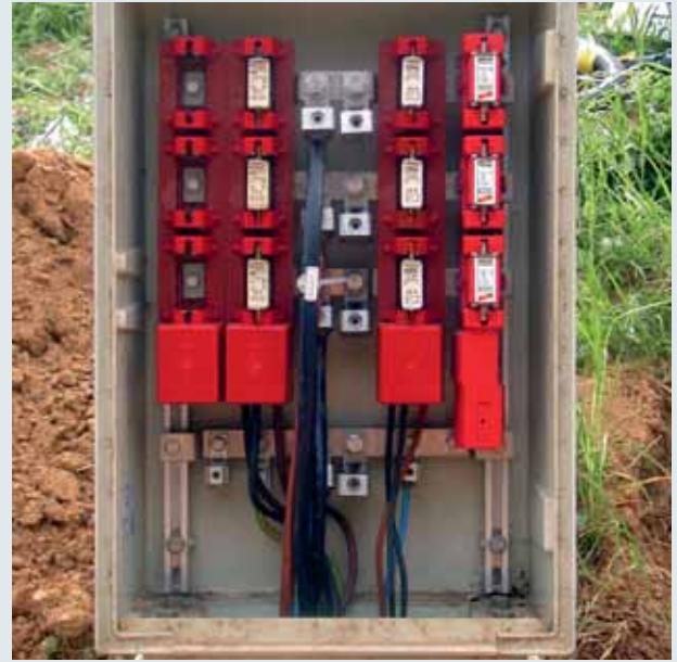
For protecting low voltage consumer's installations against surges. For installation in conformity with the lightning protection zones concept at the boundaries from O_B - 1 and higher. German patented design.
