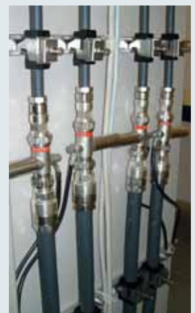
Application of quarter-wave arresters
