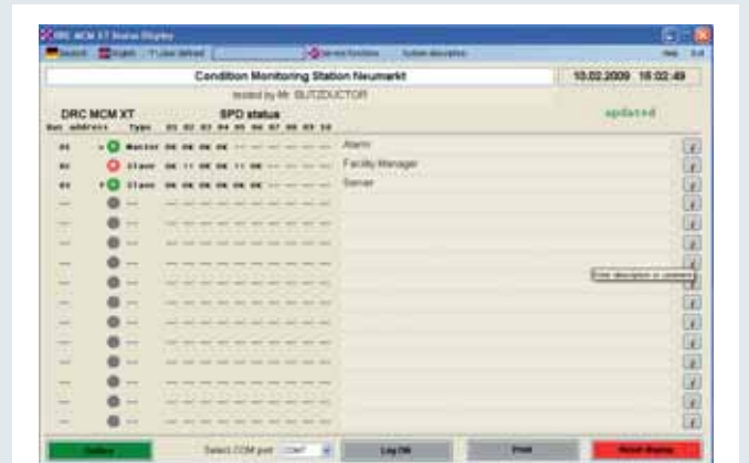
Graphical status indication of DRC MCM XT monitoring systems and of all programmed protection modules assigned to them.
