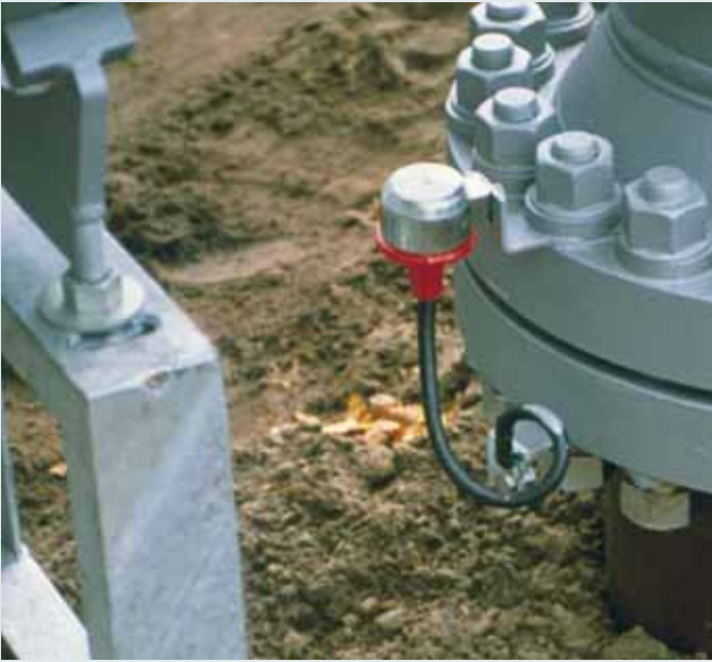
ATEX and IECEx-certified isolating spark gap for lightning equipotential bonding according to IEC 62305 with flexible conductor connection
