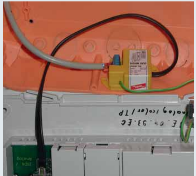
Flush-mounted surge arrester used in LAN interfaces
