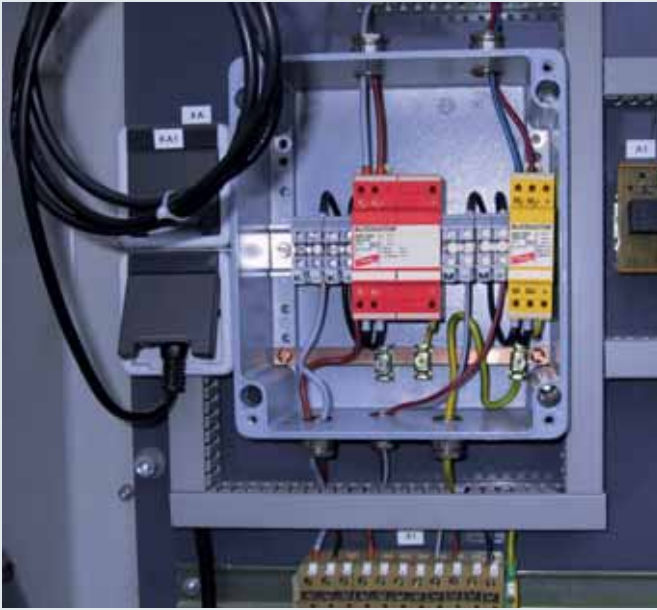
Arrester for protecting active cathodic corrosion protection systems. Integrated floating remote signalling contact (break contact) for function monitoring.
