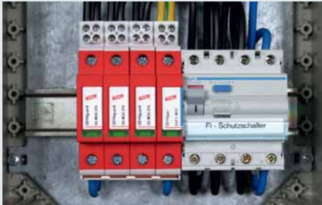
EMC-optimized feed-through wiring of lightning current and surge arresters according to IEC 60364-5-53 by means of STAK 2X16
