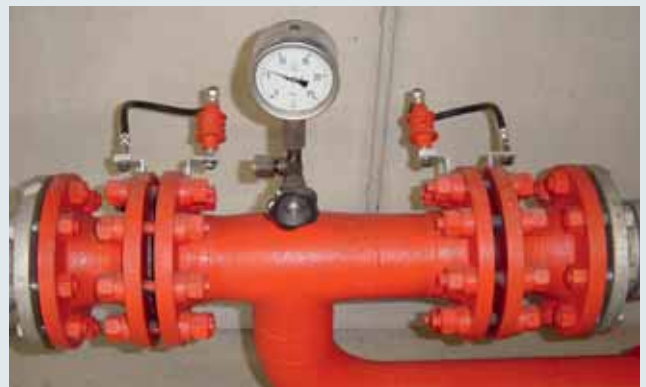
EXFS 100 KU types are enclosed by a moisture-proof plastic sheath and are therefore ideally suited for underground installation on insulating couplings.
