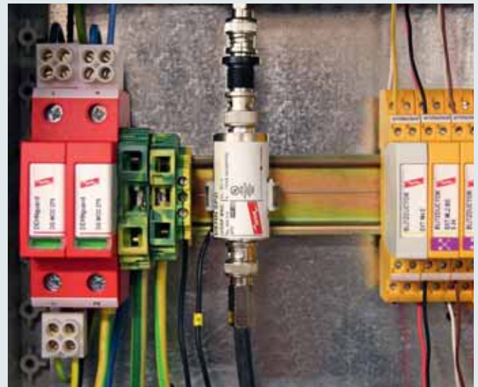
Surge arrester designed as cable adapter for protecting coaxial systems such as video and camera systems from potential damage.
