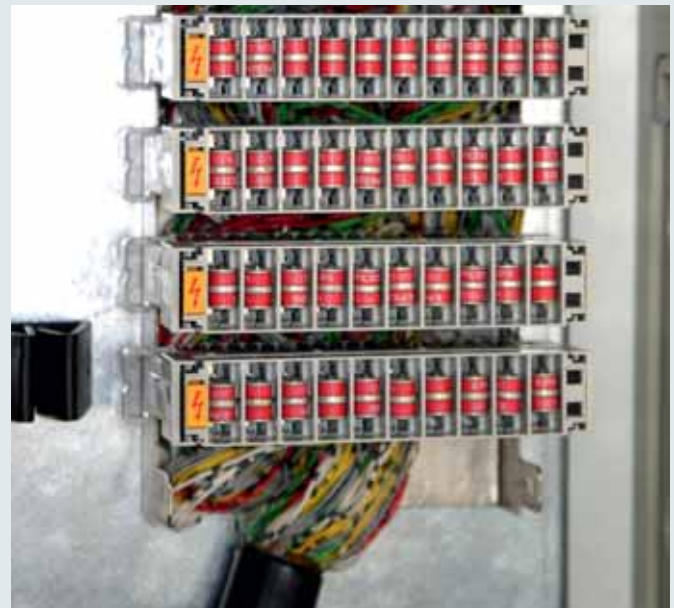
Pluggable arresters for use in LSA systems of 2/10 type. For use as protection block for 10 pairs with individually replaceable protection elements.
