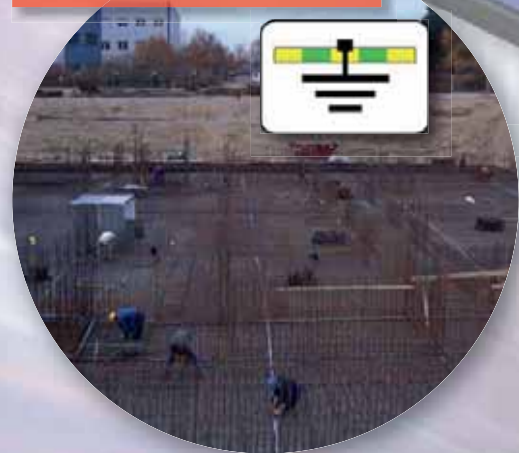
DEHN Earthing Tool - Page 20 Calculation of the length of the earth electrodes in accordance with EN 62305-3
