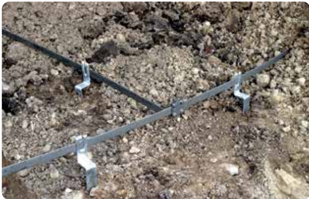
Application of the spacer with cross unit
