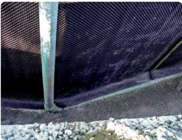
Application of the dimpled sheets
