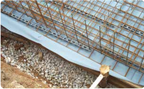
Foil under the foundation plate
