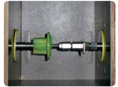
Wall bushing with formwork installation
