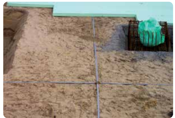
Detail view of ring earth electrode
