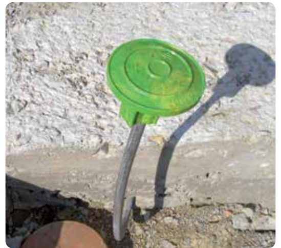
Protective cap on terminal lug
