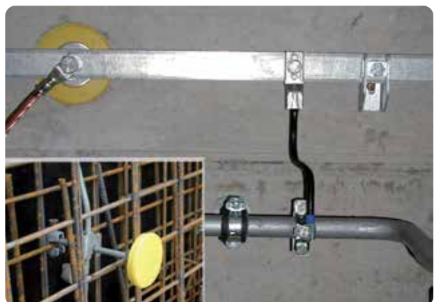
Application of the fixed earthing terminal
