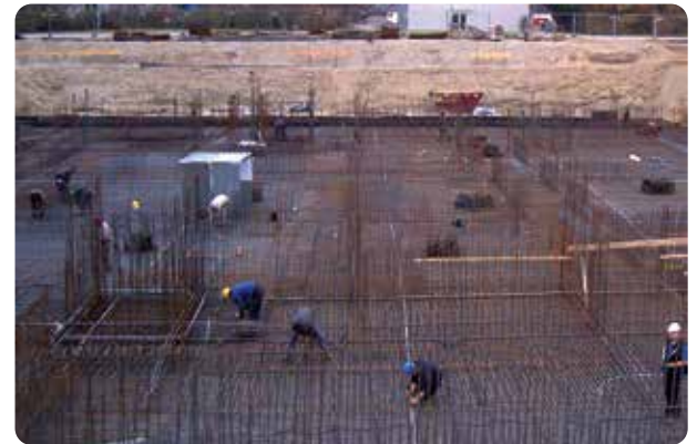
Foundation earth electrode with meshes
