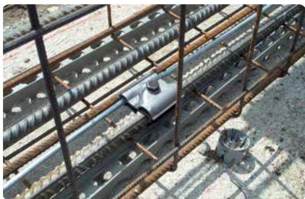
Application of the MAXI MV Clamp
