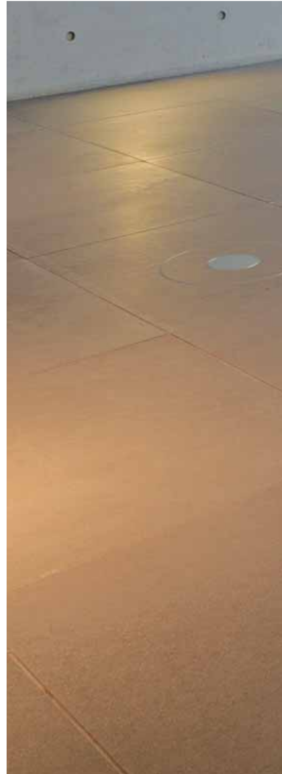
Left: square height-adjustable cassette with cable outlet
