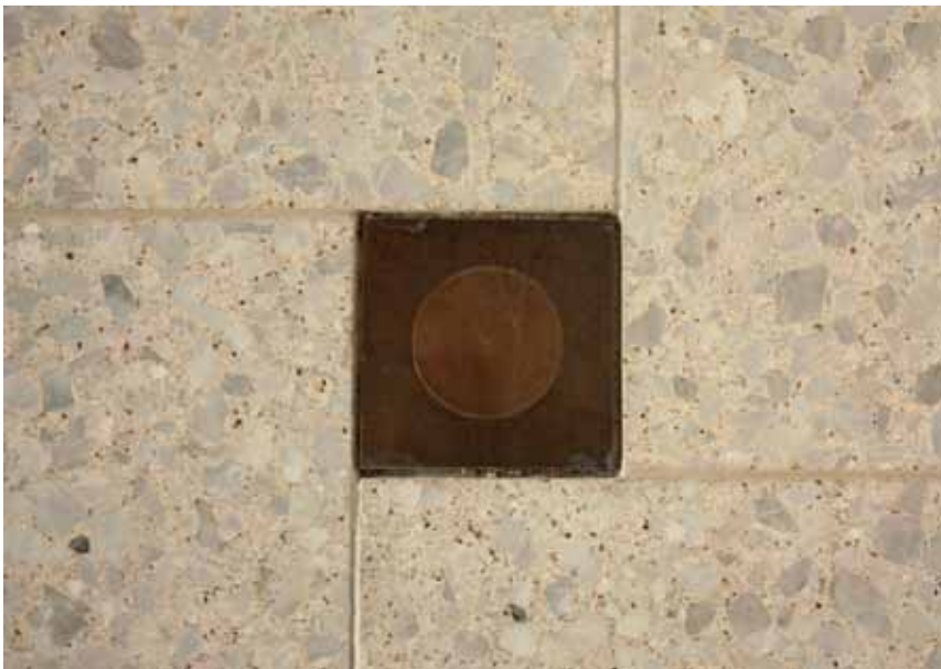
Cable outlet with tube body at the New Museum in Berlin
