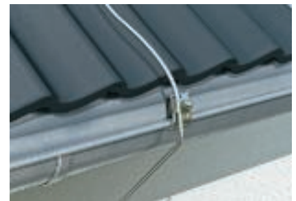
Conductor, connected with gutter clamp
