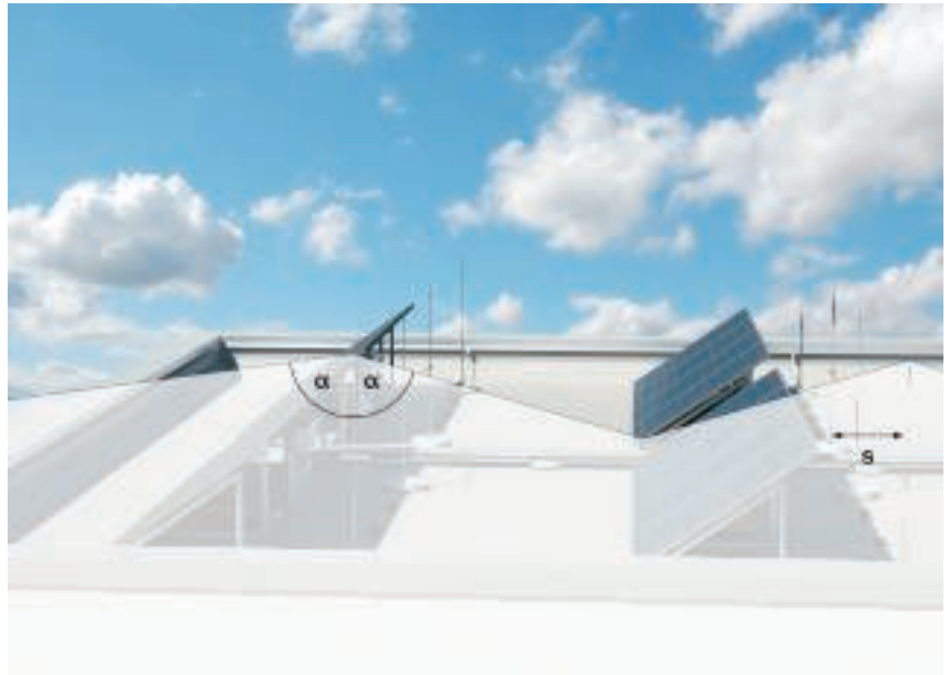
\alpha^\circ = lightning protection angle, s = separating distance
